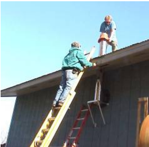
Extending the stack so it vents above the roof
