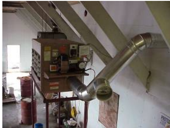
Installation complete! Note the chimney stack
