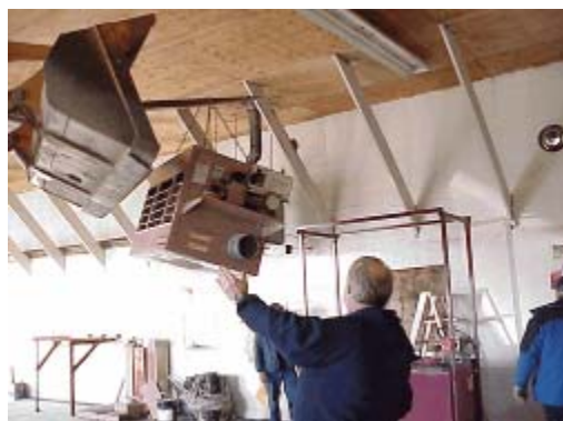
Heavy equipment being used to lift heater unit onto the used oil burner
