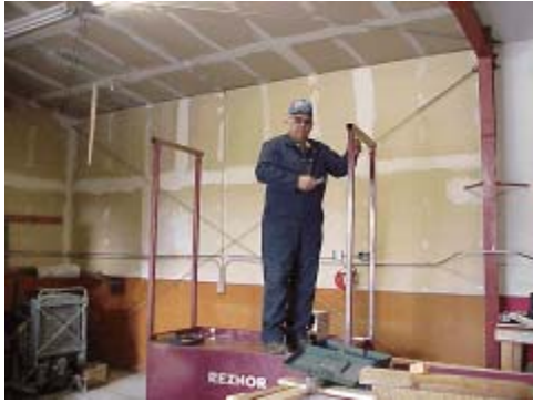
Starting the installation of a used oil burner at Goodnews Bay (Dennis Lundine, DEC )
